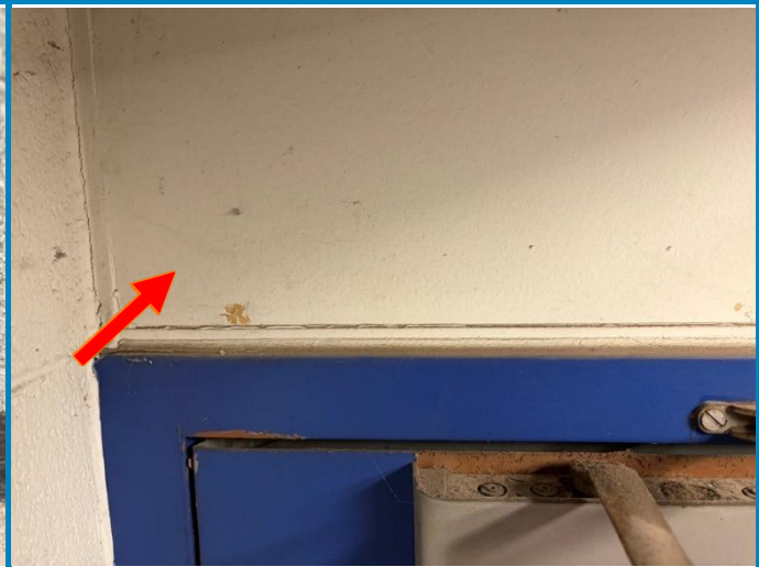
Photo 6: View of a wood panel, without joint compound, observed above the door within the 2 nd floor entrance vestibule (Loc# 48777).
