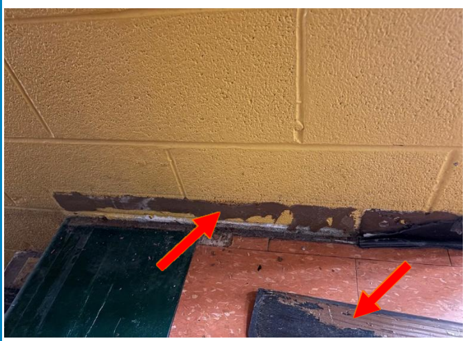
Photo 2: View of a portion of the non-asbestos-containing brown baseboard mastic (see arrows) observed within the basement stage area (Loc# 73832)
