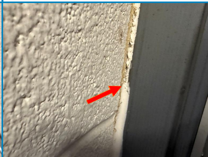
Photo 12: View of newly applied white caulking on the double door (see arrow), with no secondary layer observed beneath, observed within the 2 nd floor entrance vestibule (Loc# 48777).
