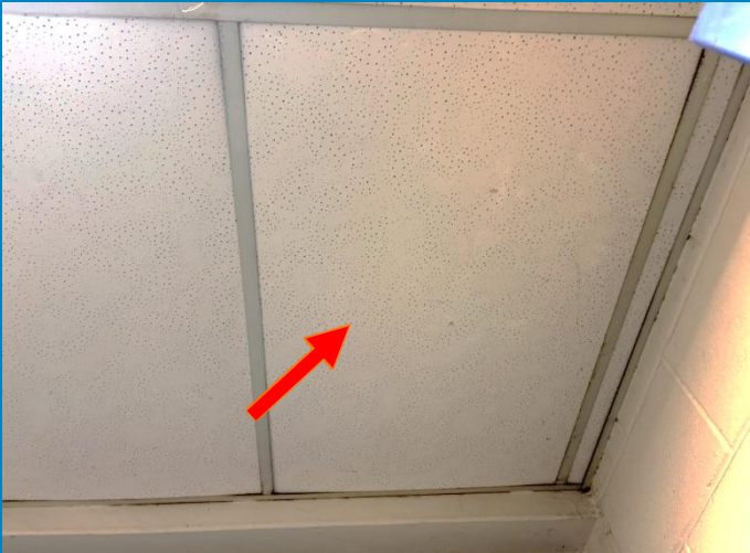
Photo 4: View of the asbestos-containing 2'x4' small holes and pinholes in circular pattern (see arrow) observed within the 2 nd floor entrance vestibule (Loc# 48777)
