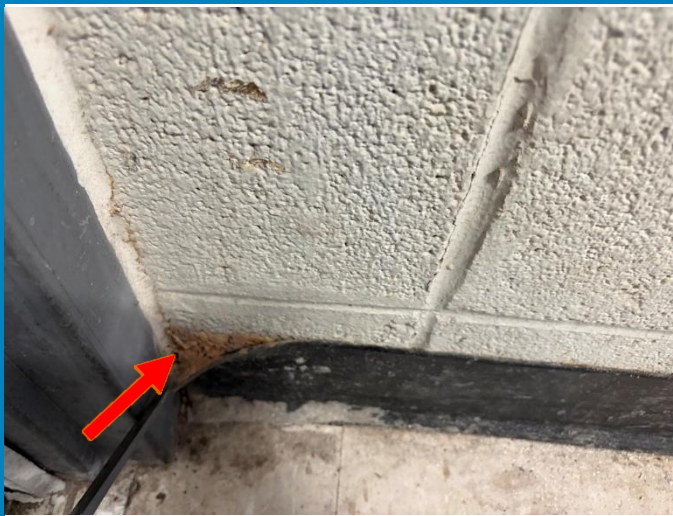
Photo 5: View of a portion of the non-asbestos-containing yellow baseboard mastic (see arrow) observed within the 2 nd floor entrance vestibule (Loc# 48777)
