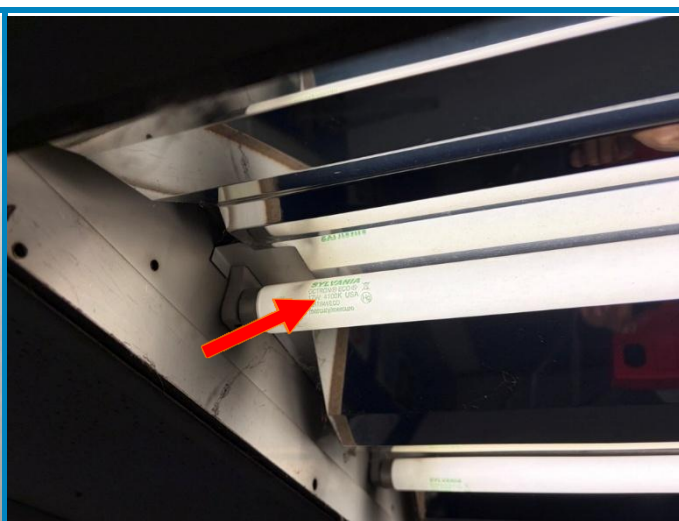
Photo 14: View of the mercury containing light tubes observed in the basement storage room (Loc# 73834) and the 2 nd floor entrance vestibule (Loc# 48777).
