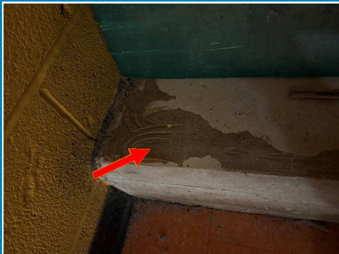
Photo 3: View of the non-asbestos-containing brown mastic (see arrow) observed under green vinyl sheet flooring on the stair within the basement stage area (Loc# 73832).
