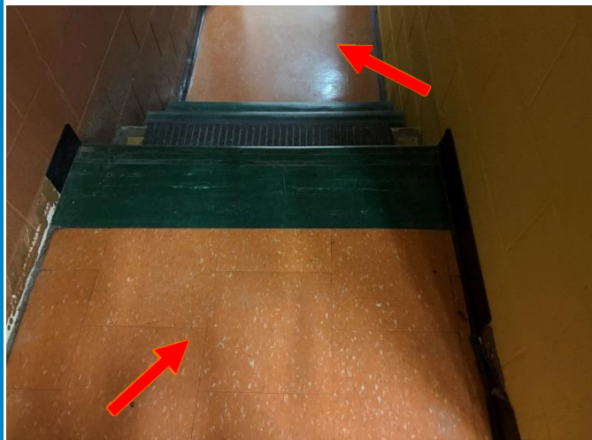
Photo 1: View of the asbestos-containing 12"x12" orange with dark orange, light orange and white flecks vinyl floor tiles (see arrows), with underlying non-asbestos-containing brown floor mastic observed within the basement stage area (Loc# 73832)
