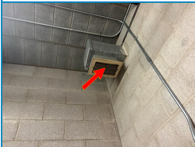
Photo 11: View of the existing exhaust ductwork (see arrow), which is planned to be relocated, appearing uninsulated with no caulking or tar observed in the basement storage room (Loc# 73834).
