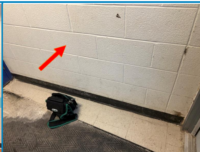
Photo 10: View of a concrete block (see arrow) with asbestos-containing white block sealant, along with white paint on the concrete wall that was determined to contain a lead concentration exceeding the 0.009% limit as outlined in the federal surface coating regulation, observed within the 2 nd floor entrance vestibule (Loc# 48777).
